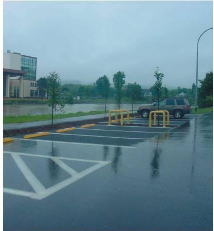
Using Porous Asphalt and CU-Structural Soil®
